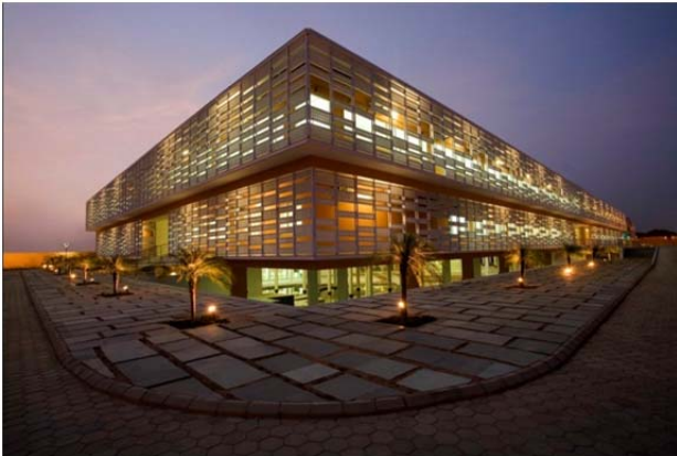
Fig. 1: Façade of building showing Jalli work.
